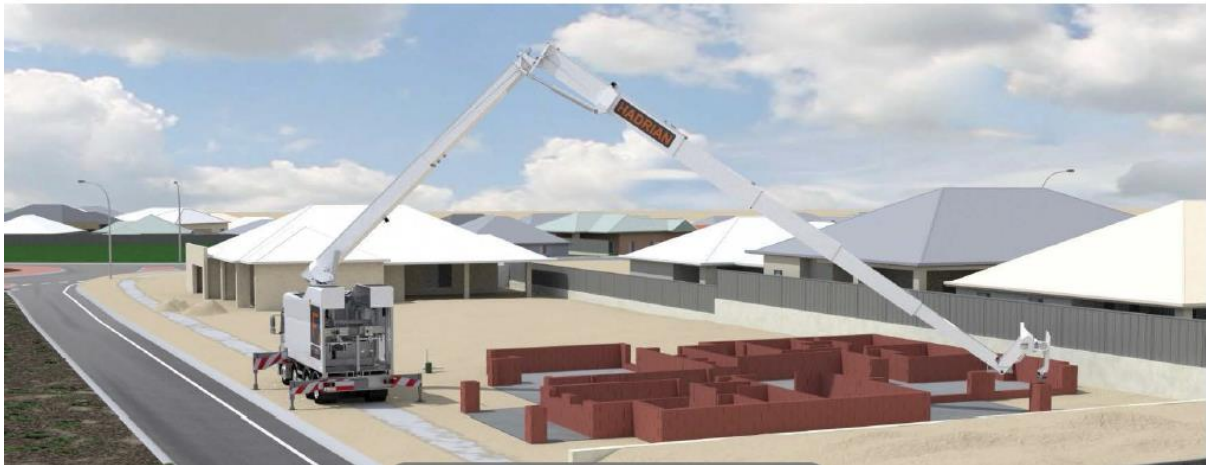
Figure 3: Illustration (computer simulation) of Hadrian X Construction Robot
